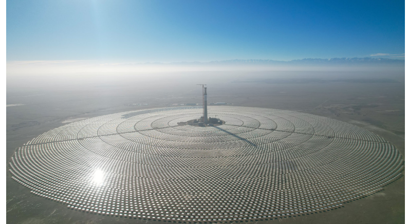
The solar field glowing in the sun
