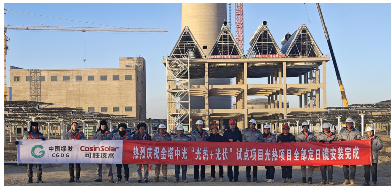
All heliostats have been installed
